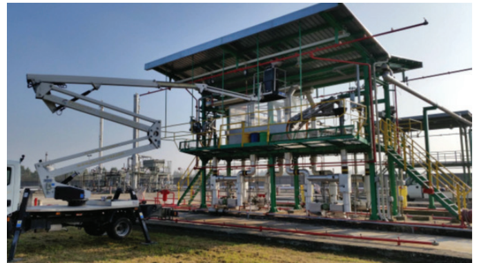
Example of installation of RAIL.
